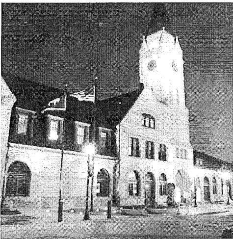
The former Union Pacific depot glows in nighttime lighting in Cheyenne, Wyo. PHOTO PROVIDED
